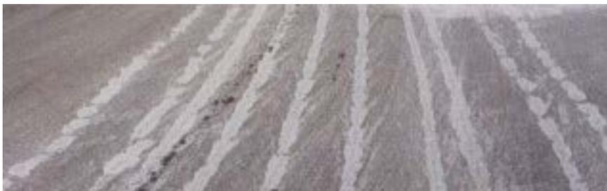
Example of wet/dry anti-icing spread pattern
