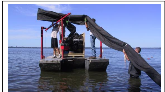
Fig. 4. Boom wall being unloaded from a barge, June 2012. (Photo: R. Lathrop, WDNR).
