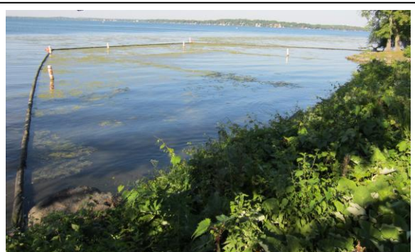
Fig. 10. Deflector boom system deployed at Olin Beach in 2012 showing aquatic plants and filamentous algae growing inside and outside the boom system. (Photo: R. Lathrop, WDNR)
